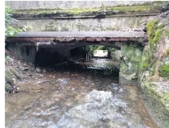
Figure 67: Aval traversée RD3 (01/21)
