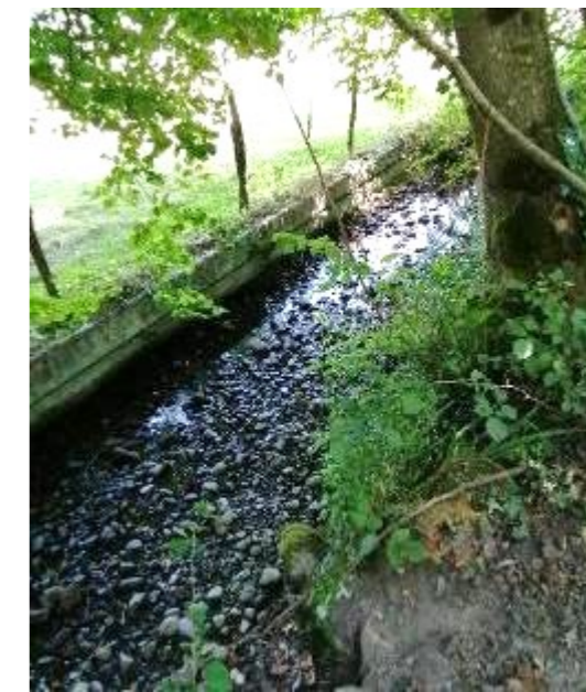
Figure 34: Protection de berge - Aval Vieux Marigny (07/20)
