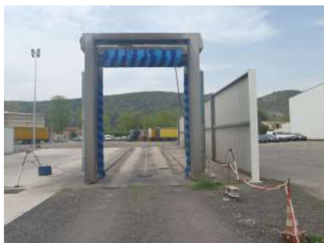
Station de lavage
