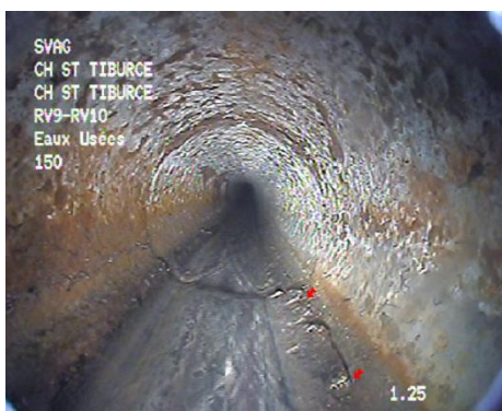
Corrosion + Fissure
