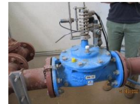
Vanne anti-intrusion
