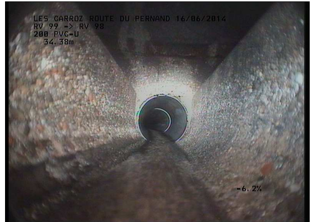
Photo: 9_6A, MPEG #: 160614_1, 00:03:06 34,68m, Fin de l'inspection RV 99 SCERCL
