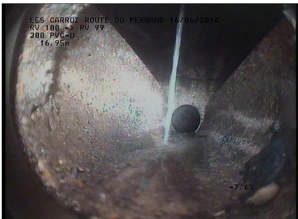
Photo: 8_6A, MPEG #: 160614_1, 00:03:28 17,5m, Fin de l'inspection RV 100 SCERCL
