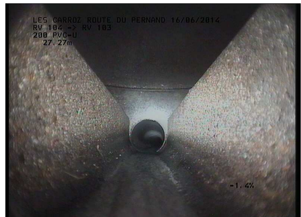
Photo: 4_8A, MPEG #: 160614_1, 00:04:02 27,76m, Fin de l'inspection RV 103
