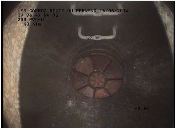
Photo: 12_6B, MPEG #: 160614_1, 00:04:20 48,41m, Fin de l'inspection RV 96 SCERCL
