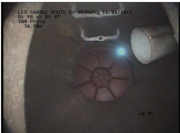
Photo: 10_5B, MPEG #: 160614_1, 00:03:28 36,9m, Fin de l'inspection RV 98 SCERCL
