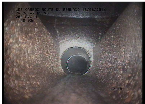
Photo: 12_6A, MPEG #: 160614_1, 00:04:20 48,41m, Fin de l'inspection RV 96 SCERCL
