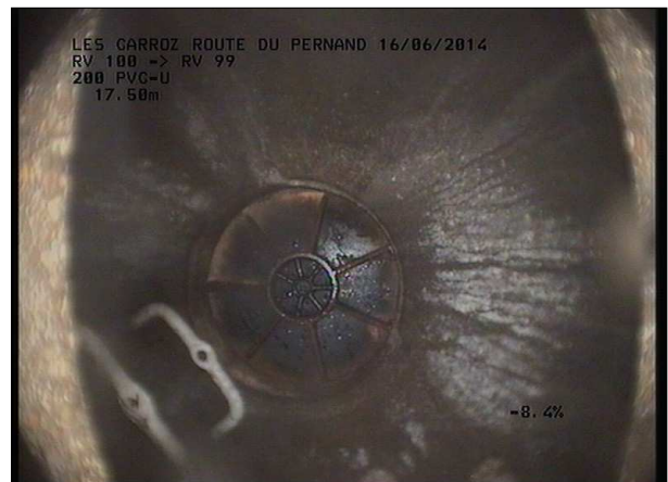
Photo: 8_6B, MPEG #: 160614_1, 00:03:28 17,5m, Fin de l'inspection RV 100 SCERCL
