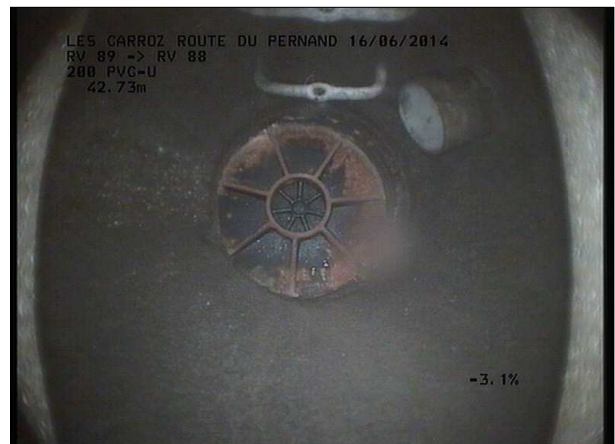
Photo: 19_7B, MPEG #: 160614_1, 00:04:23 42,73m, Fin de l'inspection RV 80 SCERCL
