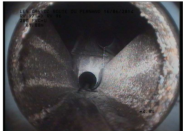
Photo: 11_2A, MPEG #: 160614_1, 00:03:56 62,45m, Fin de l'inspection RV 97 SCERCL
