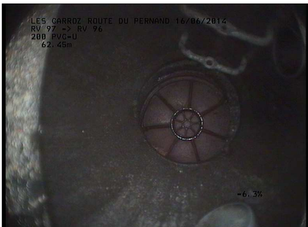
Photo: 11_2B, MPEG #: 160614_1, 00:03:56 62,45m, Fin de l'inspection RV 97 SCERCL
