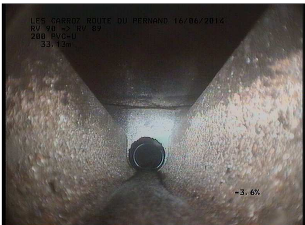
Photo: 18_3A, MPEG #: 160614_1, 00:02:52 33,58m, Fin de l'inspection RV 81 SCERCL
