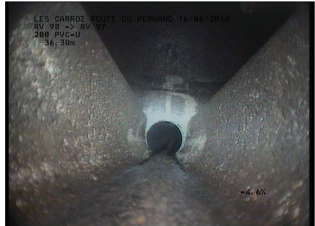
Photo: 10_5A, MPEG #: 160614_1, 00:03:28 36,9m, Fin de l'inspection RV 98 SCERCL
