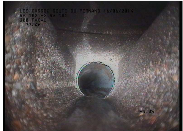
Photo: 6_2A, MPEG #: 160614_1, 00:02:32 33,62m, Fin de l'inspection RV 101
