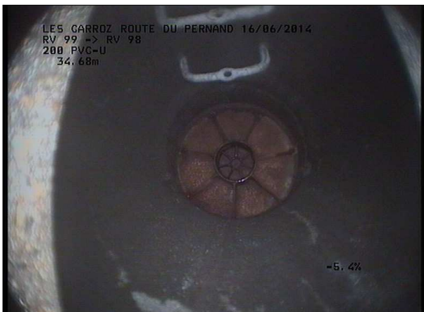
Photo: 9_6B, MPEG #: 160614_1, 00:03:06 34,68m, Fin de l'inspection RV 99 SCERCL
