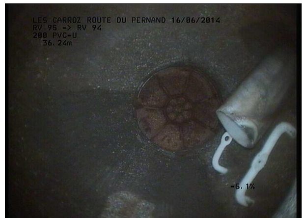
Photo: 13_6B, MPEG #: 160614_1, 00:03:43 36,24m, Fin de l'inspection RV 94 SERCL
