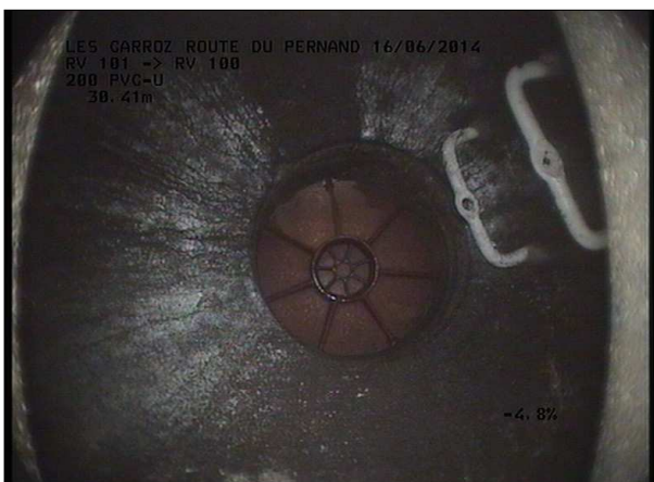
Photo: 7_2B, MPEG #: 160614_1, 00:02:30 30,41m, Fin de l'inspection RV 101 SCERCL
