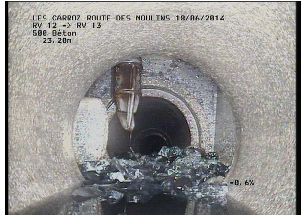
Photo: 12_2A, MPEG #: 180614_1, 00:07:41 24,49m, Fin de l'inspection R 247
