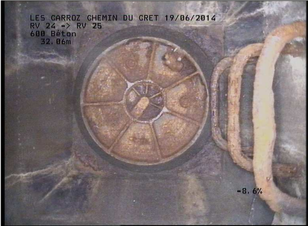
Photo: 24_5B, MPEG #: 180614_1, 00:02:52 32,06m, Fin de l'inspection R 897
