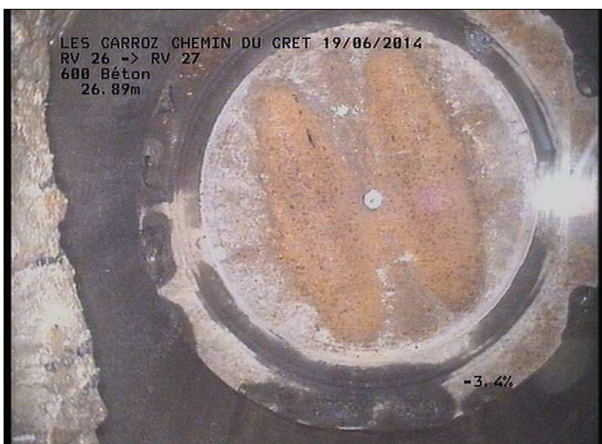
Photo: 26_2B, MPEG #: 180614_1, 00:01:40 26,89m, Fin de l'inspection R 554
