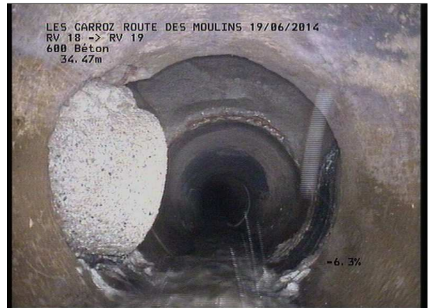
Photo: 18_2A, MPEG #: 180614_1, 00:01:56 34,47m, Fin de l'inspection R 943
