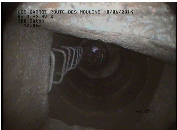
Photo: 3_8B, MPEG #: 180614_1, 00:03:03 17,06m, Fin de l'inspection R 287
