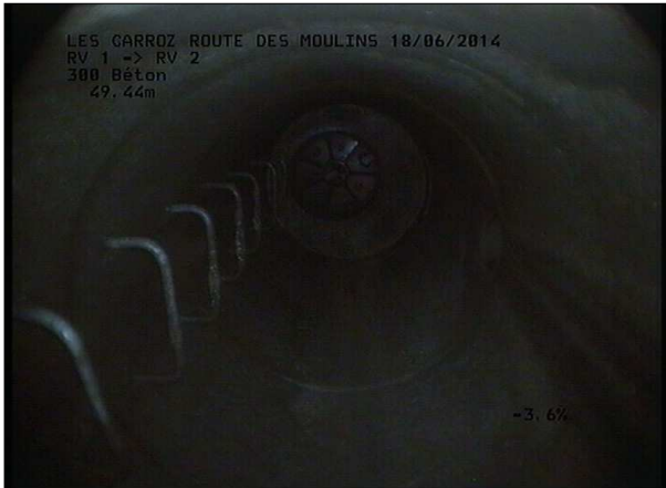
Photo: 1_18B, MPEG #: 180614_1, 00:07:50 49,44m, Fin de l'inspection R 293
