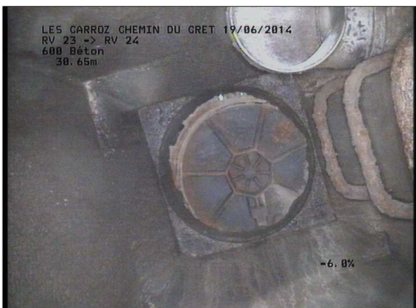
Photo: 23_2B, MPEG #: 180614_1, 00:02:00 30,65m, Fin de l'inspection R 904
