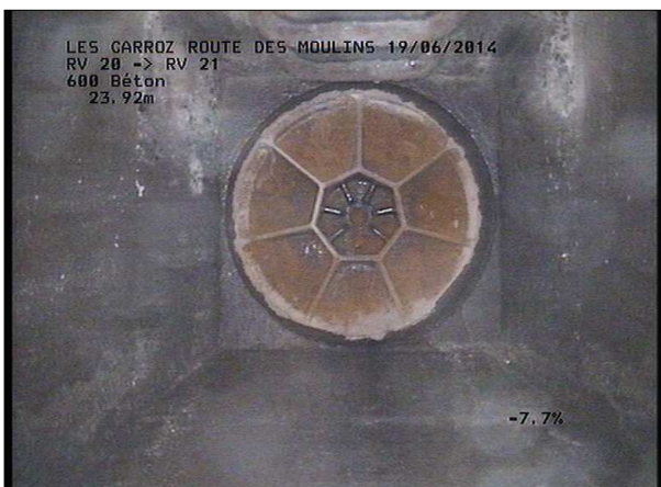
Photo: 20_2B, MPEG #: 180614_1, 00:01:21 23,92m, Fin de l'inspection R 921
