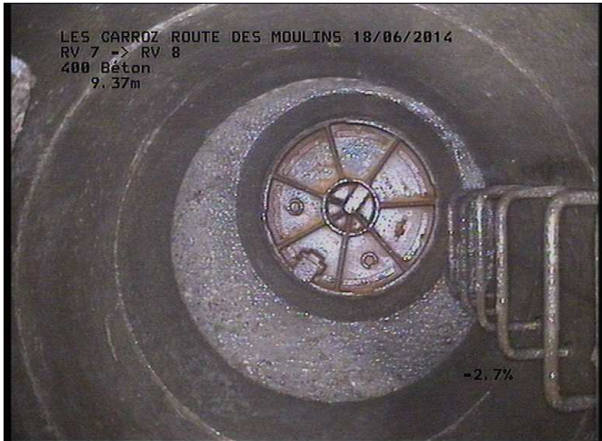
Photo: 7_7B, MPEG #: 180614_1, 00:03:19 9,37m, Fin de l'inspection R 280
