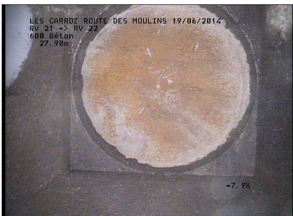
Photo: 21_6B, MPEG #: 180614_1, 00:03:05 27,98m, Fin de l'inspection R 914
