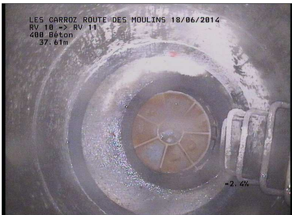
Photo: 10_6B, MPEG #: 180614_1, 00:05:15 37,61m, Fin de l'inspection R 264
