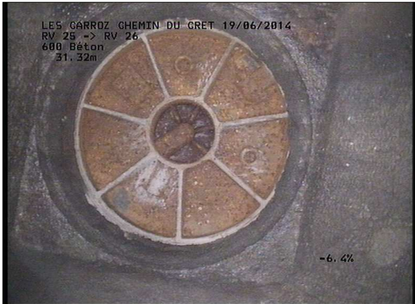
Photo: 25_5B, MPEG #: 180614_1, 00:04:39 31,32m, Fin de l'inspection R 579
