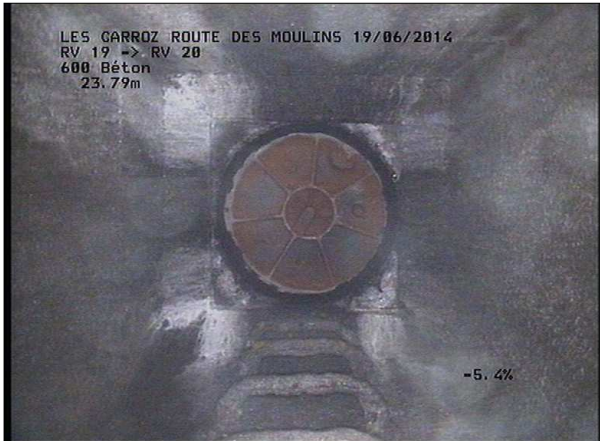
Photo: 19_2B, MPEG #: 180614_1, 00:01:16 23,79m, Fin de l'inspection R 924
