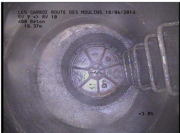
Photo: 9_4B, MPEG #: 180614_1, 00:03:01 18,37m, Fin de l'inspection R 273
