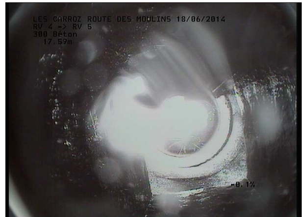
Photo: 4_6B, MPEG #: 180614_1, 00:02:04 17,59m, Fin de l'inspection R 284
