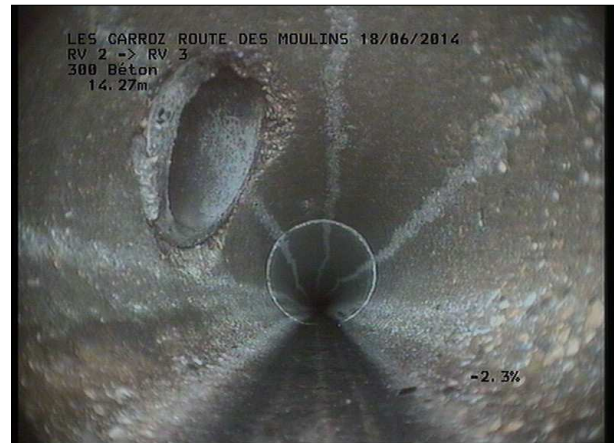
Photo: 2_6A, MPEG #: 180614_1, 00:02:14 14,67m, Raccordement direct à 10 h.
