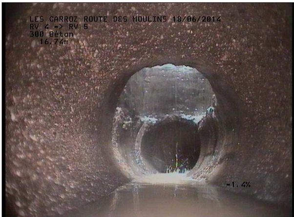
Photo: 4_6A, MPEG #: 180614_1, 00:02:04 17,59m, Fin de l'inspection R 284
