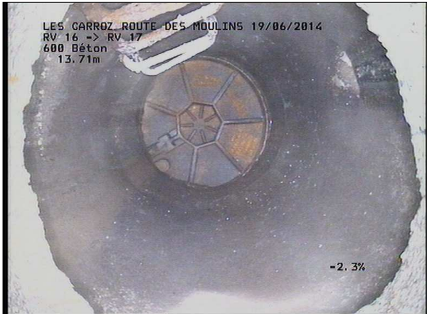
Photo: 16_3B, MPEG #: 180614_1, 00:01:15 13,71m, Fin de l'inspection R 957
