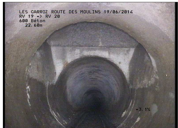
Photo: 19_2A, MPEG #: 180614_1, 00:01:16 23,79m, Fin de l'inspection R 924
