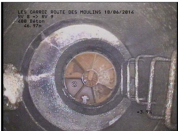
Photo: 8_10B, MPEG #: 180614_1, 00:06:45 46,97m, Fin de l'inspection R 274
