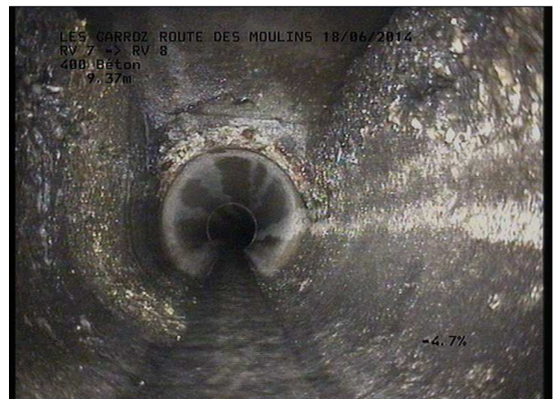
Photo: 7_7A, MPEG #: 180614_1, 00:03:19 9,37m, Fin de l'inspection R 280
