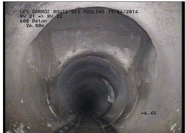
Photo: 21_6A, MPEG #: 180614_1, 00:03:05 27,98m, Fin de l'inspection R 914
