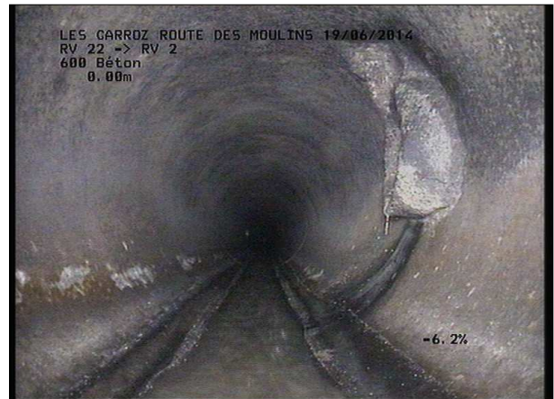
Photo: 22_2A, MPEG #: 180614_1, 00:00:05 1,37m, Raccordement direct à 02 h.
