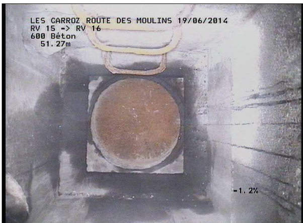
Photo: 15_4B, MPEG #: 180614_1, 00:03:44 51,27m, Fin de l'inspection R 958
