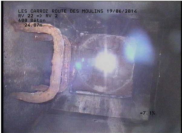
Photo: 22_5B, MPEG #: 180614_1, 00:02:06 24,87m, Fin de l'inspection R 905
