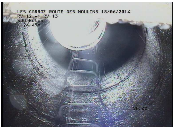
Photo: 12_2B, MPEG #: 180614_1, 00:07:41 24,49m, Fin de l'inspection R 247
