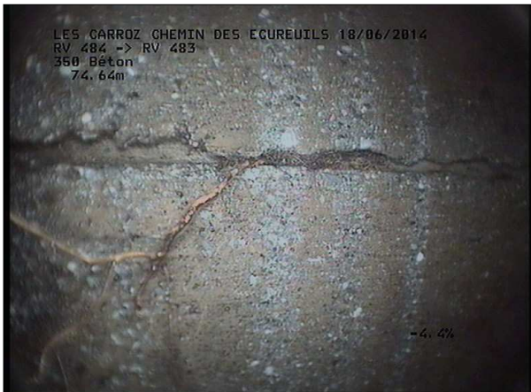
Photo: 23_17B, MPEG #: 160614_1, 00:11:53 74,64m, Radicelles à 09 h.
