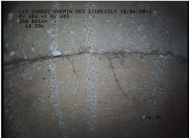
Photo: 23_13B, MPEG #: 160614_1, 00:09:23 62,33m, Radicelles à 10 h.
