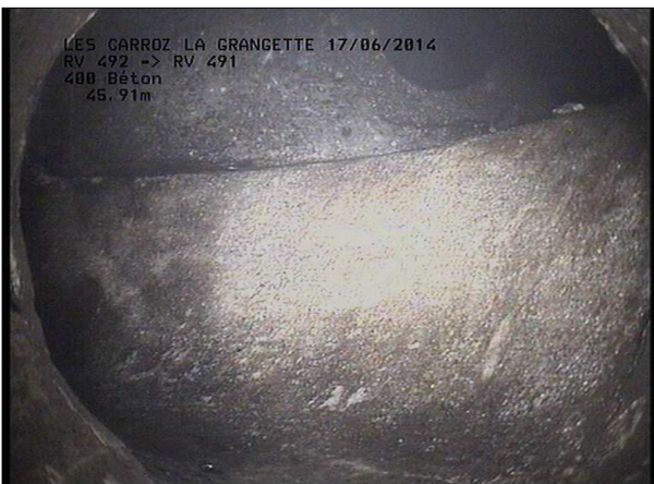
Photo: 9_22A, MPEG #: 160614_1, 00:10:47 46,42m, Fin de l'inspection RV 491
