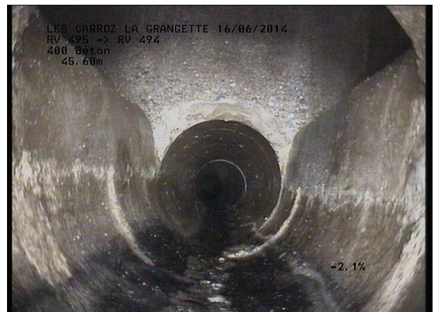
Photo: 6_13A, MPEG #: 160614_1, 00:08:19 46,26m, Fin de l'inspection RV 494
