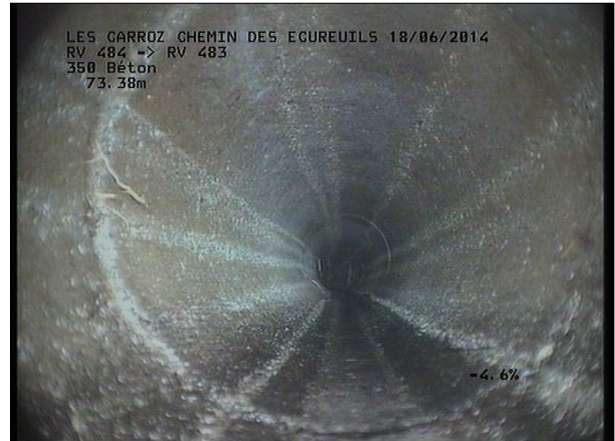
Photo: 23_16A, MPEG #: 160614_1, 00:11:17 73,58m, Radicelles à 09 h.
