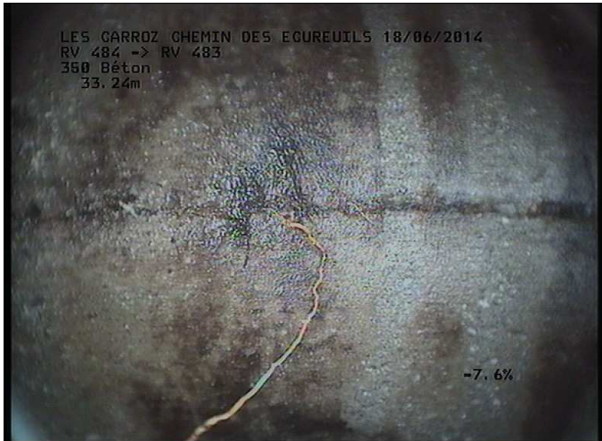
Photo: 23_7B, MPEG #: 160614_1, 00:04:13 33,24m, Radicelles à 11 h.
