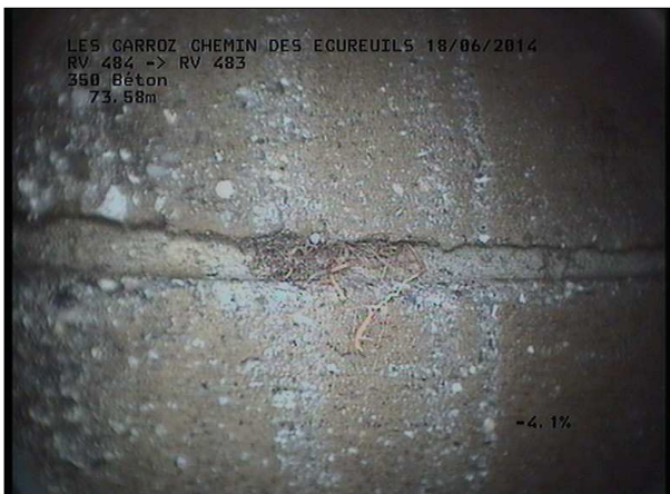
Photo: 23_16B, MPEG #: 160614_1, 00:11:17 73,58m, Radicelles à 09 h.
