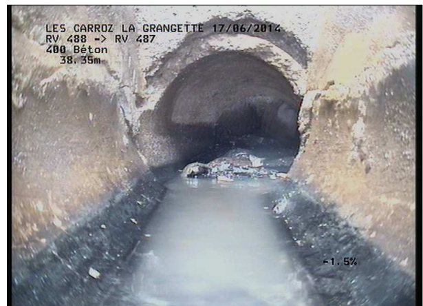
Photo: 13_12A, MPEG #: 160614_1, 00:06:56 38,78m, Fin de l'inspection RV 487
