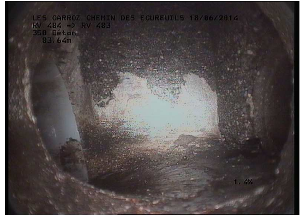
Photo: 23_22A, MPEG #: 160614_1, 00:14:25 83,64m, Fin de l'inspection RV 480 SCERCL
