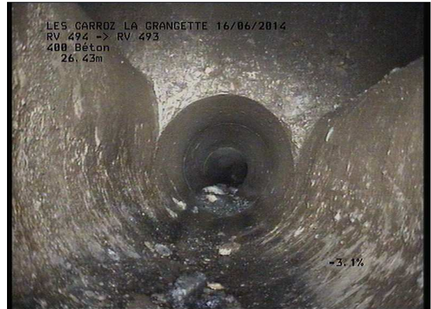
Photo: 7_10A, MPEG #: 160614_1, 00:06:12 26,43m, Fin de l'inspection RV 493
