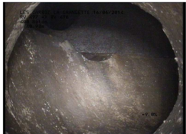
Photo: 4_17A, MPEG #: 160614_1, 00:10:07 41,53m, Fin de l'inspection RV 496
