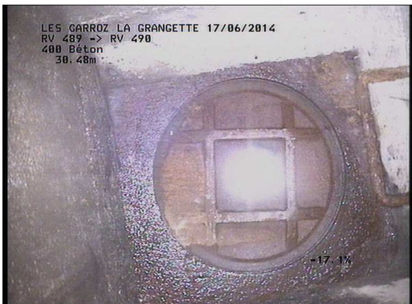
Photo: 11_10B, MPEG #: 160614_1, 00:08:50 30,48m, Fin de l'inspection RV 489 SCERCL
