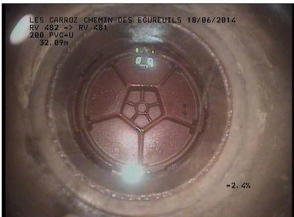
Photo: 26_2B, MPEG #: 160614_1, 00:02:21 32,09m, Fin de l'inspection RV 469 SCERCL
