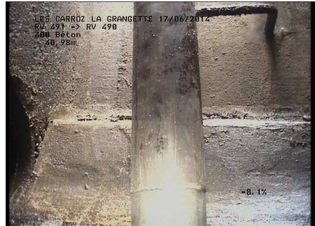
Photo: 10_23A, MPEG #: 160614_1, 00:10:23 41,57m, Fin de l'inspection RV 489 SCERCL
