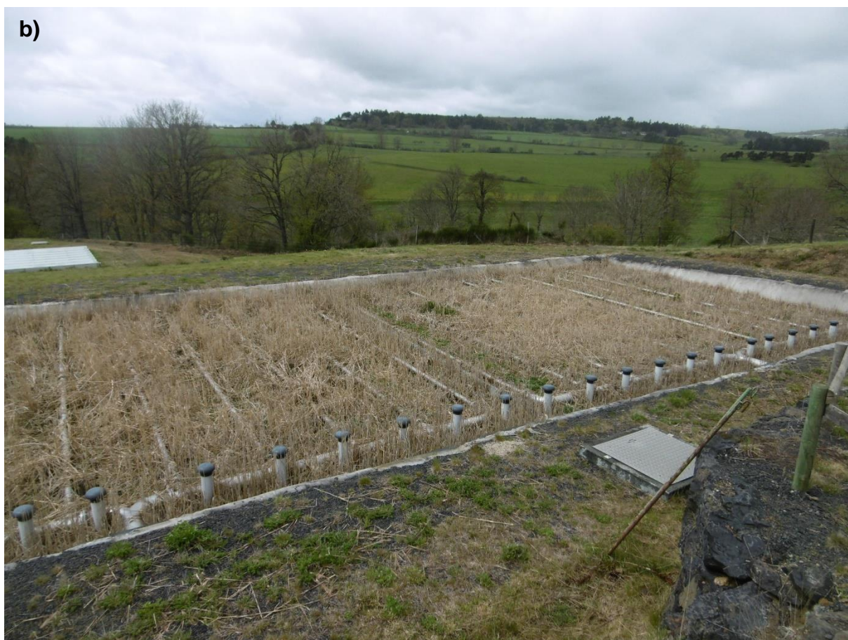
Fig. 3. 16.a) Full-scale granulated apatite filter: Filter B; b) second stage of treatment wetland plant and granulated apatite filter.
