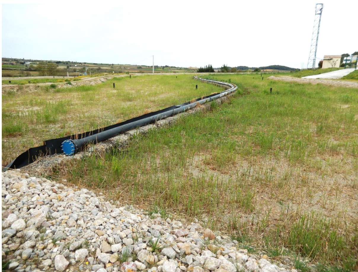
Fig. 3. 17. Second stage of the treatment wetland plant: horizontal filter + granulated apatite filter C planted with Phragmites Australis .
