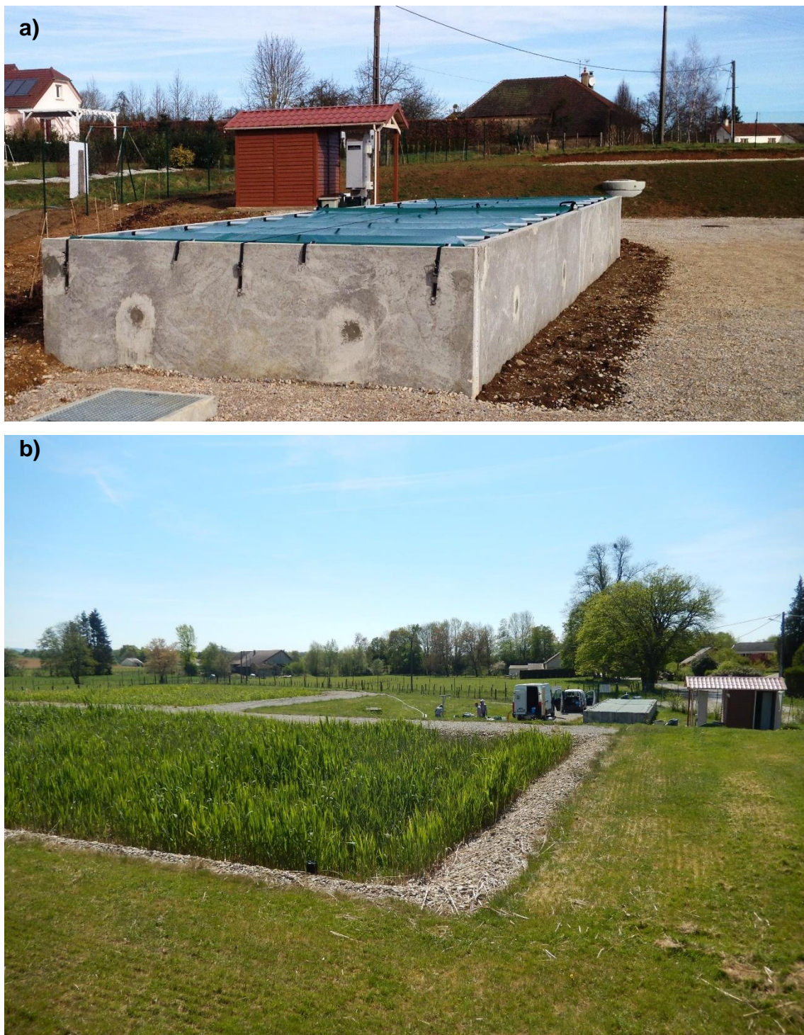
Fig. 3. 15. a) full-scaled granulated apatite filter: Filter A; b) first stage of treatment wetland plant and granulated apatite filter A.
