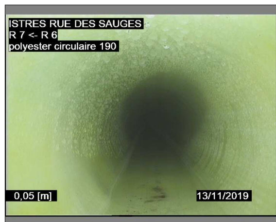
Photo: 6_1B, 00:03:04 0m, Noeud de départ, regard de visite R 7 / APRES GAINAGE
