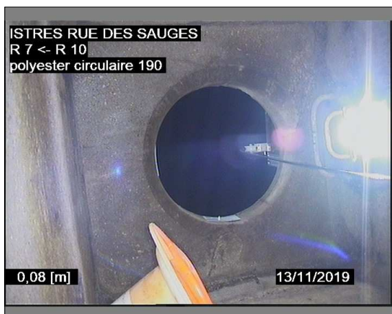
Photo: 7_1A, 00:00:00 0m, Noeud de départ, regard de visite R 7 / APRES GAINAGE
