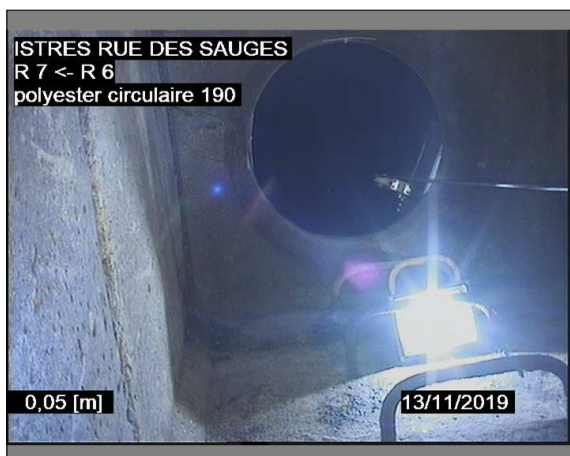
Photo: 6_1A, 00:03:04 0m, Noeud de départ, regard de visite R 7 / APRES GAINAGE
