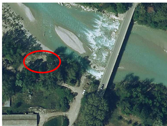
Figure 8 : Zone de base vie
