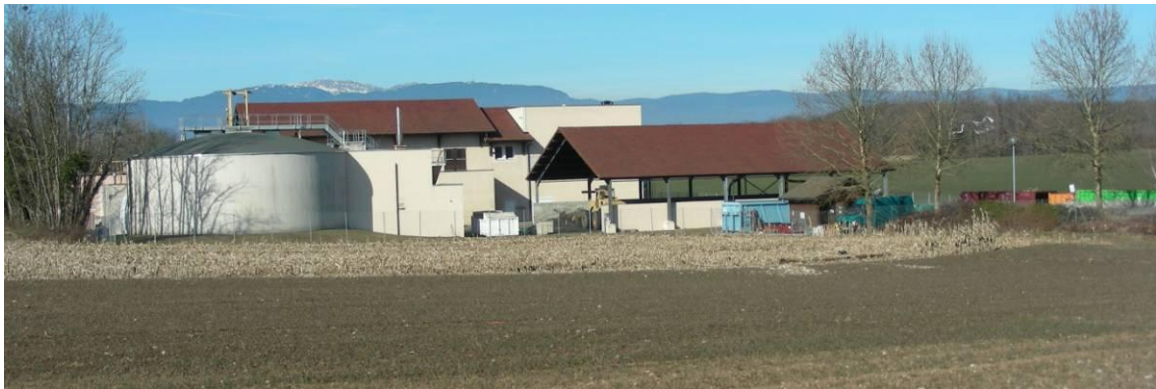
Figure 42 : Station d'épuration de Douvaine (Source: photo CIDEE)
