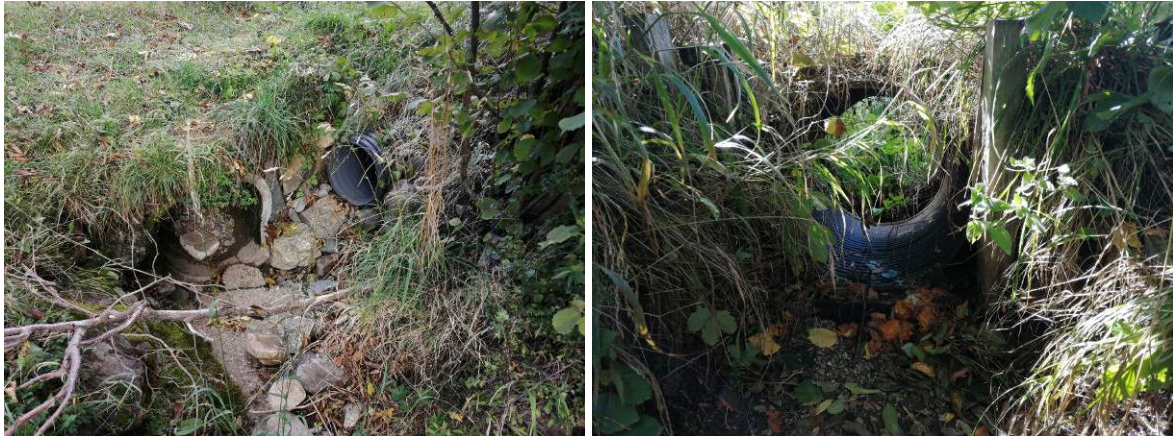
Figure 34 : Buse annelée DN400
