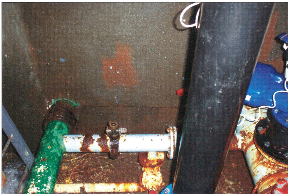
Bypass adduction/distribution
