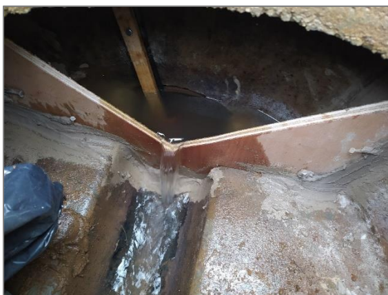
Figure 58 : Installation PDM Mont Brouilly Bourg
