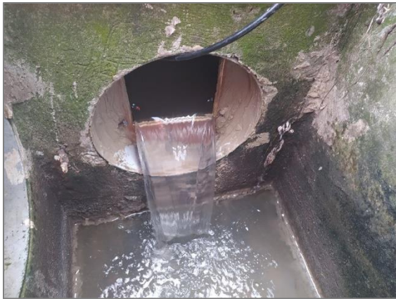
Figure 57 : Installation PDM Garanche STEP
