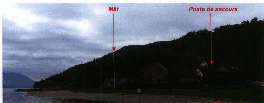
Figure 12 : Poste de secours et mât (Source: photo CIDEE)
