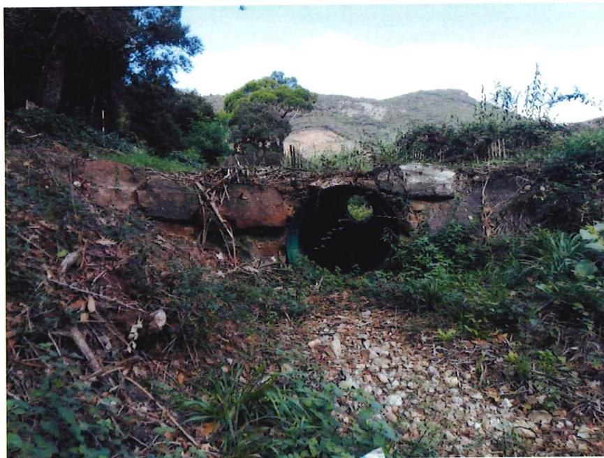
Figure 11: Ouvrage hydraulique amont (buse)
