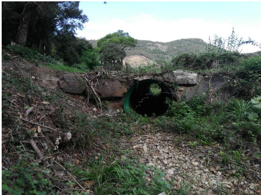
Figure 14: Ouvrage hydraulique amont (buse)
