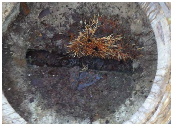
Figure 13 : Regard n°22009 – Avenue Jean Moulin
