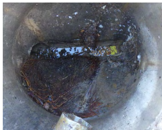
Figure 14 : Regard n°22001 – Avenue Jean Moulin
