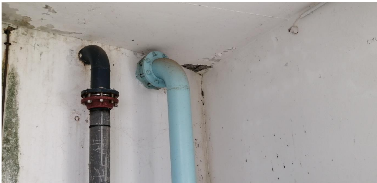
Figure 40 : Armature visible
